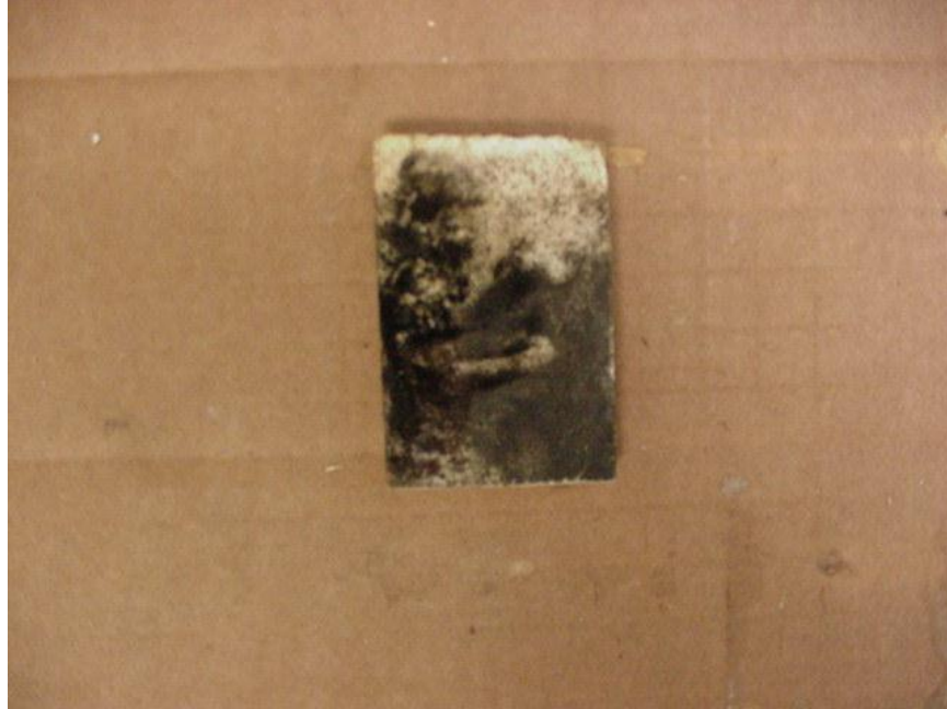
Figure 4: Painted drywall sample covered in heavy mold and stain, before CMSR.
